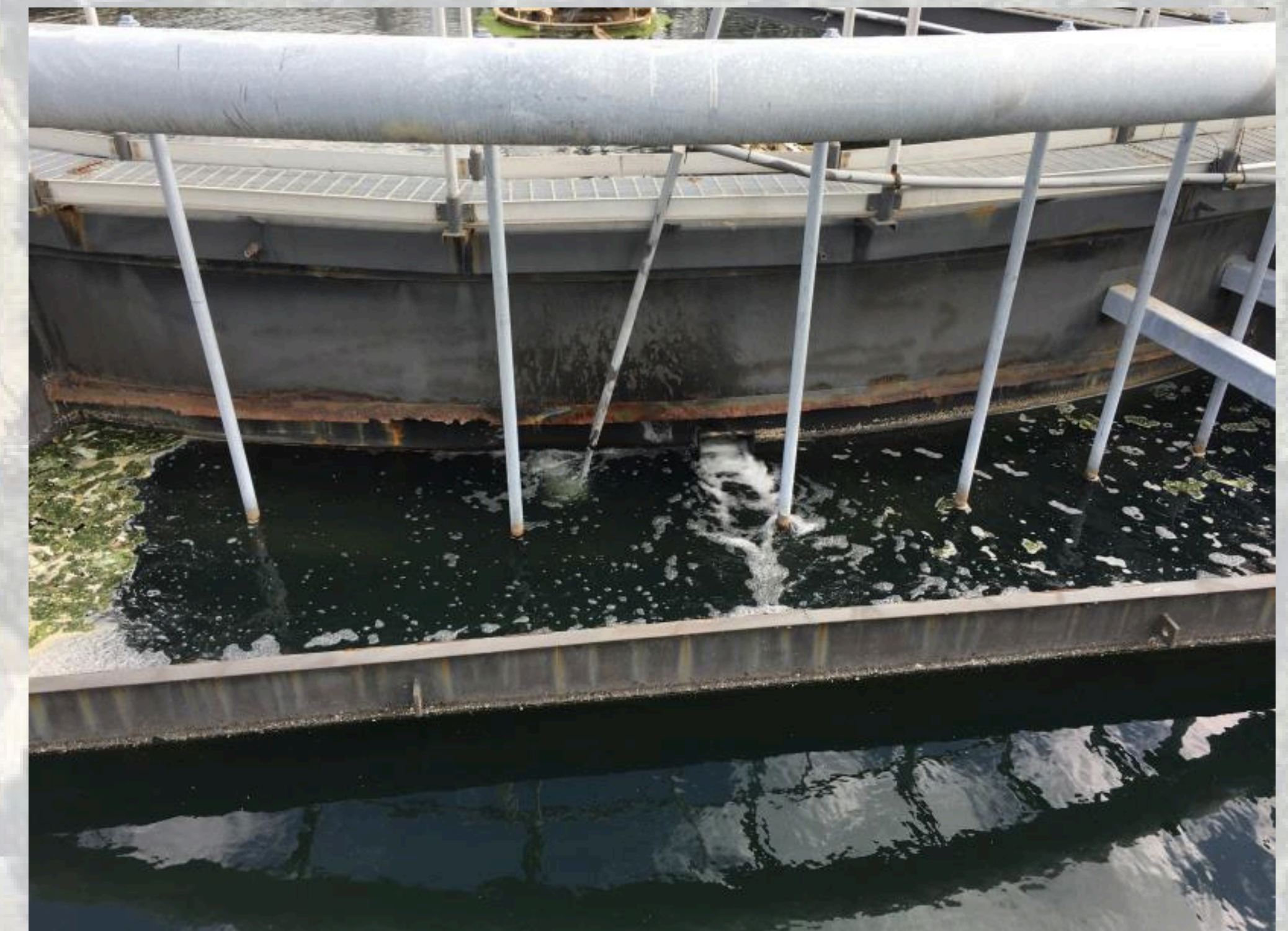
Exist Bullseye MPU Interior Wall (Corroded Stiffeners)
